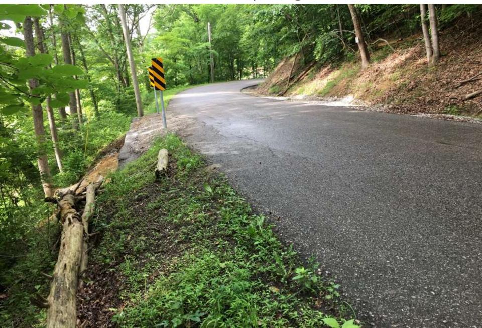
Ditch blocked by sediment from crumbling steep bank
